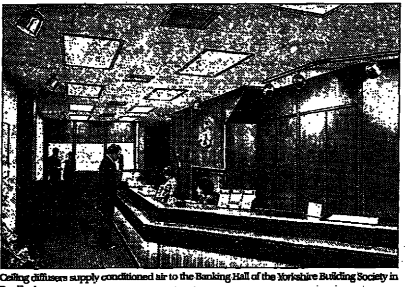
Ceiling diffusers supply conditioned air to the Banking Hall of the Yorkshire Building Society in Bradford.
